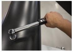
TIP! It can sometimes be a bit tricky to get all the holes to line up. To facilitate the assembly; start to line up one of the inner holes and tighten the beam bolt, leave it with a bit of play. Then continue with the other inner ones going around and then do the same procedure with the outer ones. When all bolts are in, tighten to 40 Nm. Recommended is also to go over the bolts with the torque wrench when the boat is in the water to make sure all bolts are properly tightened.
