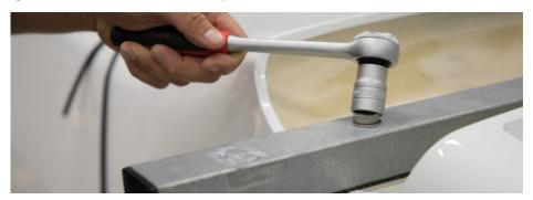
Take off the cross beam to be able to open the hatch.
